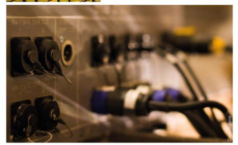
which was designed with installers Tait to allow the winch equipment to be relocated to a new, higher grid and the guides extended upward. Similarly lighting and sound facility panels on the stage galleries were terminated in panels that will allow them to be extended out to new outlets in the future.
