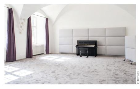
Above: To respect the protected architecture of Musikinsel Rheinau, acoustics have been improved through the use of carpet, curtains and radiator cladding, in addition to mobile and fixed panels
