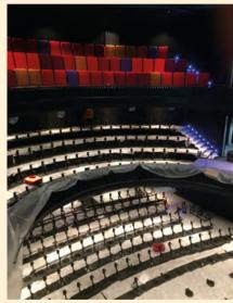
meaning some concrete levels required tiering to achieve a variable rise per row - others required a radial design to enhance the feeling of space. In the three smaller cinema rooms, a more intimate space was created through the installation of seats with arms.
