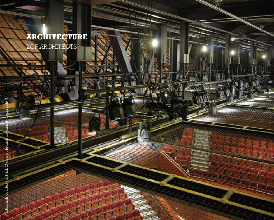
Dual-level rigging and lighting grid over the stage in the main hall
