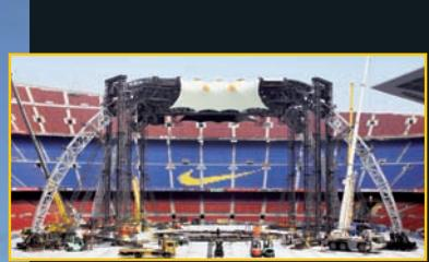
The stage for U2's 360° Tour is being constructed using Enerpac's hydraulic Synchronous Lift System
