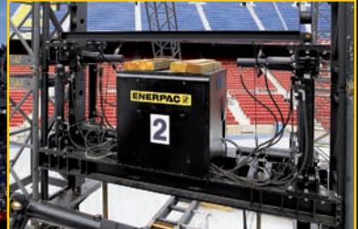
4 hydraulic units, including a pump, 4 lifting and 4 locking cylinders, climb along the temporary guide rails.
